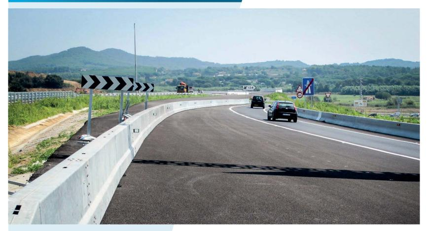
With the help of a temporary barrier the work zone can be protected for the benefit of both workforce as well as road users. Used as a lane divider for traffic, BarrierGuard 800 allows for safe traffic separation. BarrierGuard 800 offers the most appropriate solution.
